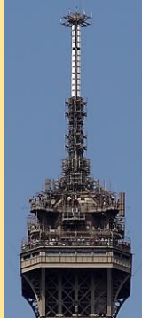
120 antennas at top of tower
